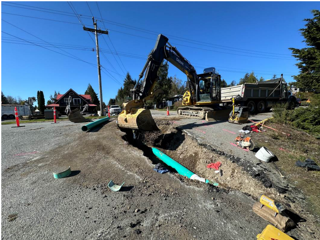
Photo #6 – Bay Street Drainage Improvements Started
