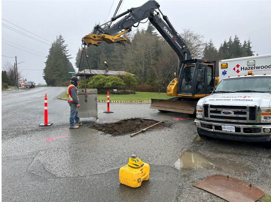
Photo #1 – New Catch Basins Installed Along Peninsula Road
