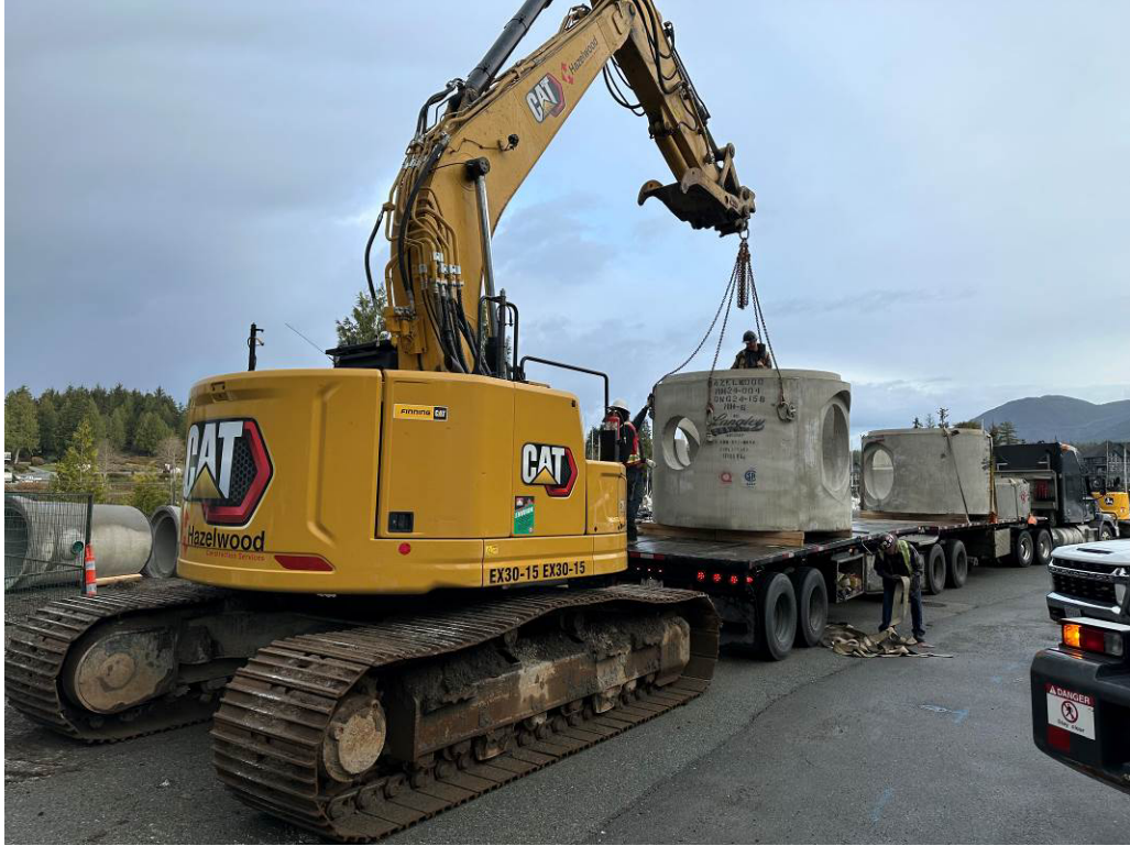
Photo #5 – DMH #6 & DMH #11 Delivered to Site
