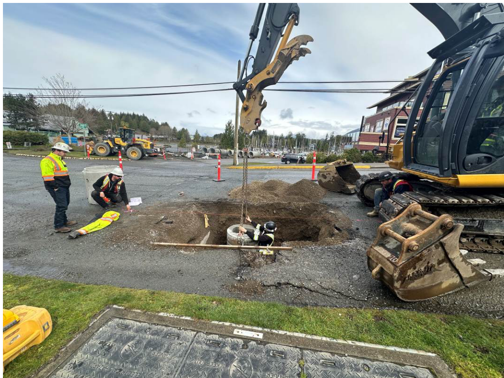
Photo #2 – New Catch Basins Installed Along Peninsula Road
