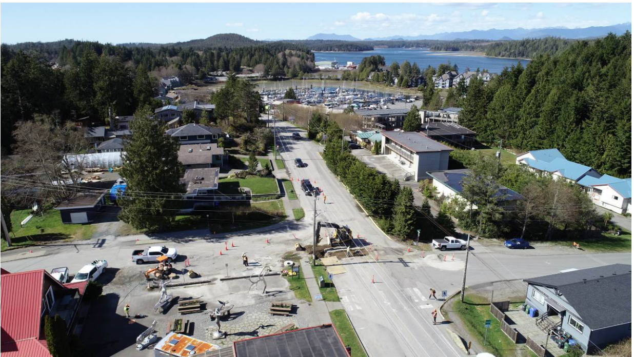
Photo #8 – Bay Street Drainage Improvements Started
