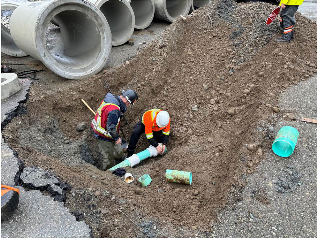
Photo #3 – Existing Catch Basins Connected to New Storm System
