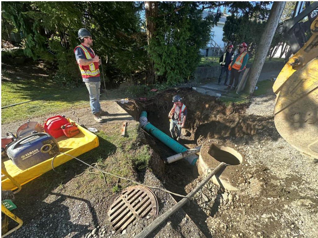
Photo #4 – Existing Catch Basins Connected to New Storm System
