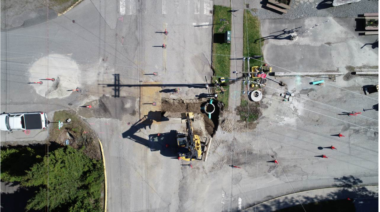
Photo #7 – Bay Street Drainage Improvements Started
