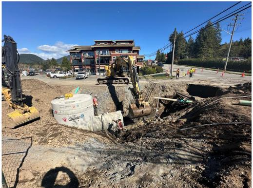
Photo #3 – Concrete Pipe Installed from DMH #11 towards DMH #6
