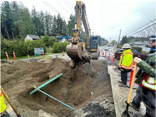
Photo #5 – Removed Existing Pipe (CSP)
