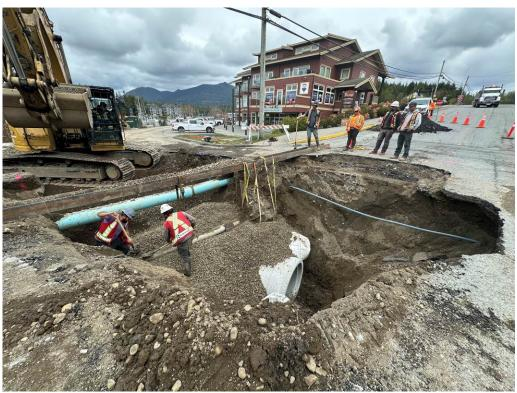
Photo #2 – Concrete Pipe Installed from DMH #11 towards DMH #6
